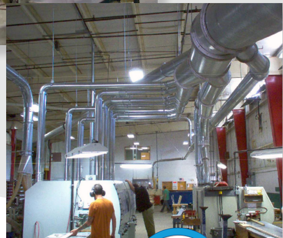
Below: After installation of Nordfab ducting.
